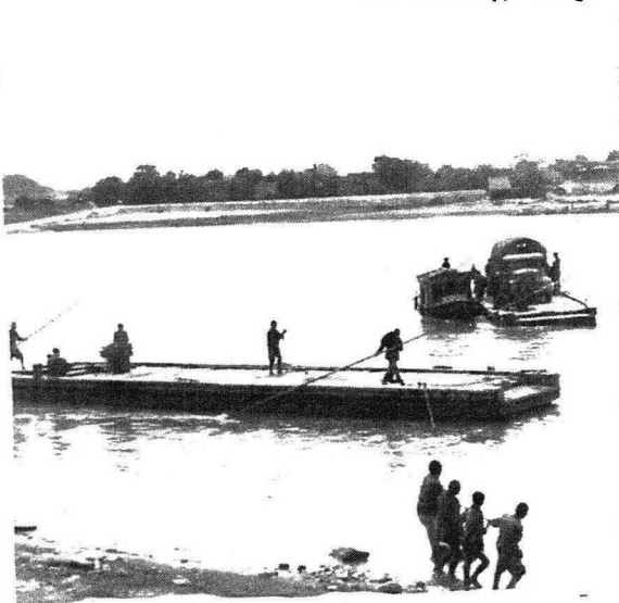
Pulling barge across river by hand
