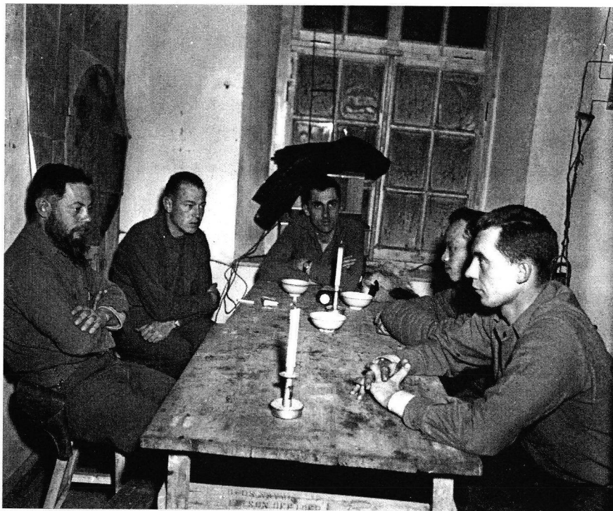
Unit 4 Mess Hall, Shenpa, Inner Mongolia 1944.
