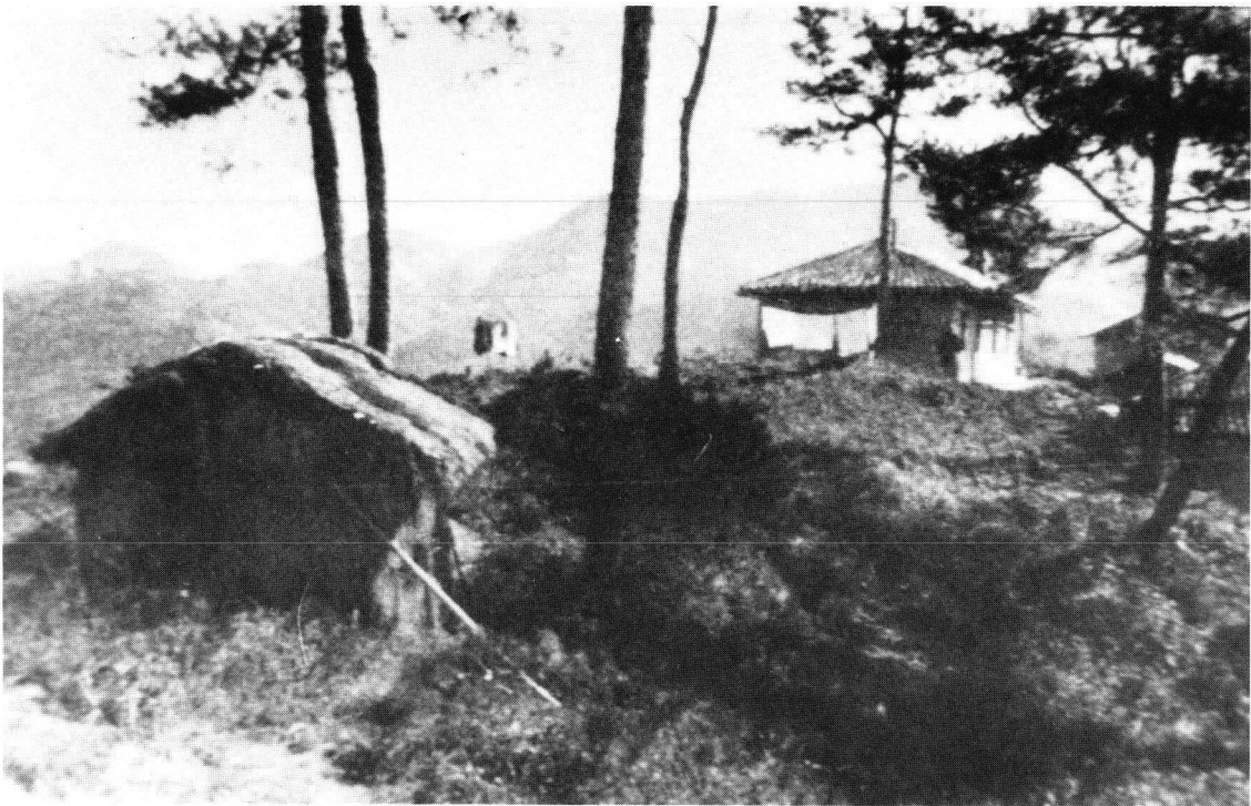
Camp 1 = Guard Shack, living quarters, radiosonde weather bldg - notice laundry line. 6-44 - 6-45
