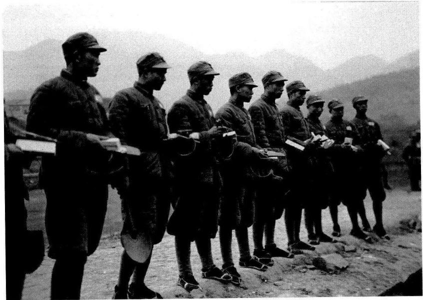
Group Leaders In Demolition Class On use and care of Explosives
