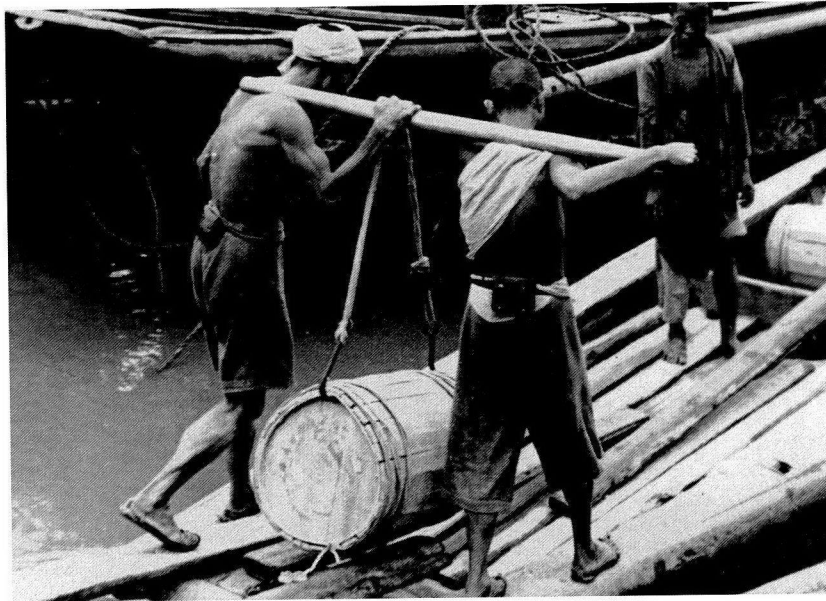
Coolies carrying a Barrel of cement
