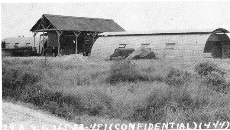
Acetylene generating plant (trailer in the middle) between two quonset huts for storage.
