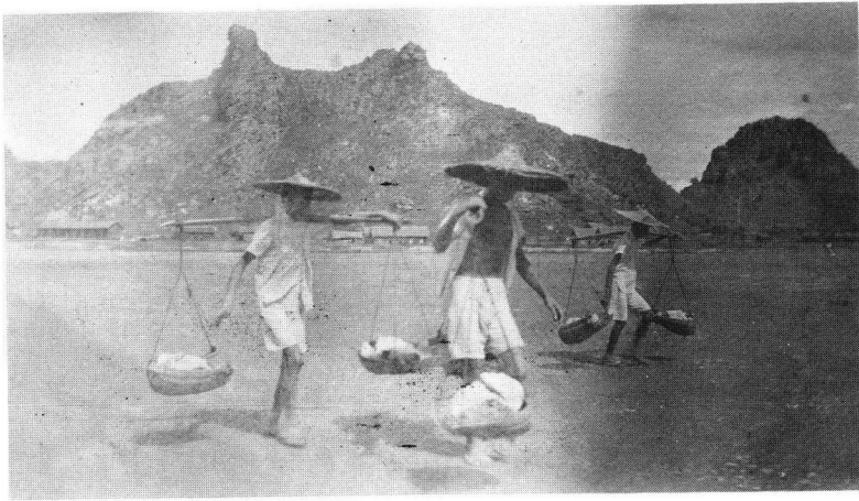
Coolies repairing airstrip in Kweilin
